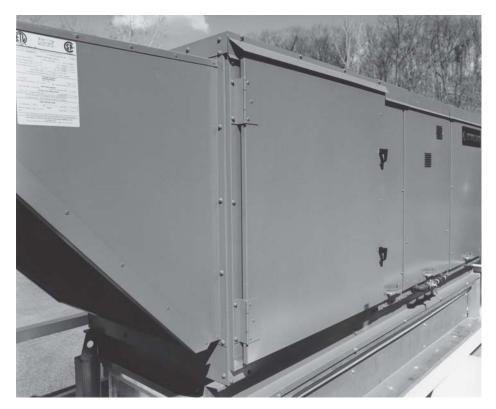
Hinged doors are mounted to the access side of the standard Blower / Filter / Damper cabinet and High CFM Filter / Damper and Blower cabinets in lieu of the standard removable access doors. The hinged doors include dual, quick opening tool-less latches and full perimeter gasketing to assure a water resistant seal. Door stops are included to guard against closure while open. The remaining Duct furnace(s) and Supply Plenum cabinets (if applicable) are supplied with a standard removable door.
